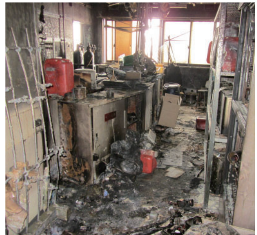
Traces of a fire of a chemical laboratory due to the shaking (in Tohoku Univ.)
